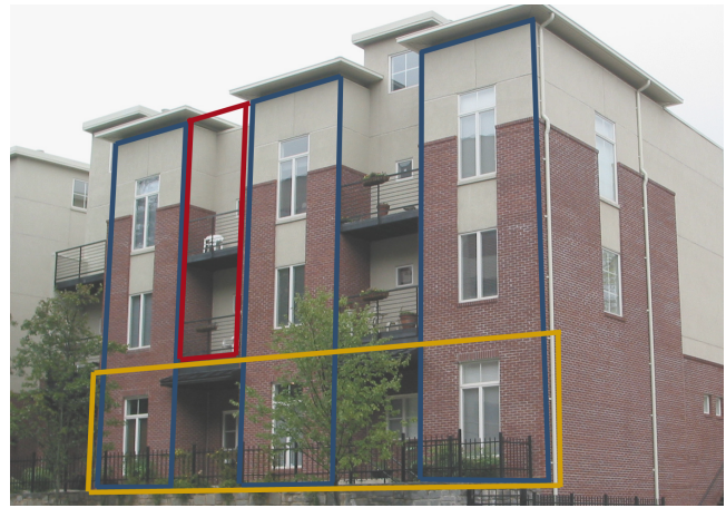
Figure 3: Photograph of a building which shows vertical coherence (balconies and material) and horizontal coherence (window styles).
