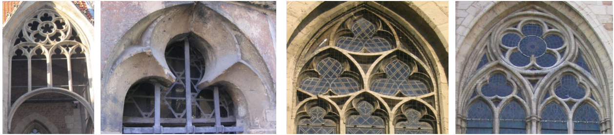
Figure 5.28: Window tracery with flat and round bars. With the flat style (a-c) the front sides of the bars form a contiguous front plane, of which the window and fillet fields are rings . This is opposed to the french style (d) with round bars. Compare the french style with the profiles created with stable extrusion in Fig. 4.80. Images are taken from the Old Town Hall (a) and the Martini church (b-d) in Braunschweig.
